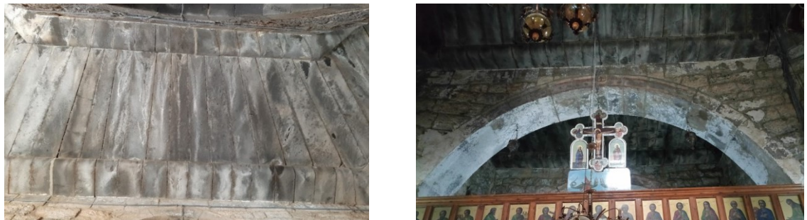
Fig. 213 The roof which is a corbelled stone slab of the south aisle, a stone arch tops the iconostasis. 2019, taken by the author.
