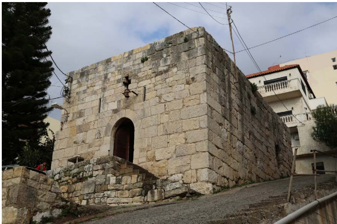
Figure 37: The spolia church of Our Lady of Qassouba - Western southern corner
