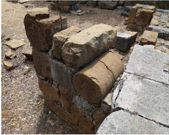
Figure 54: Re-used column drum in the Basilica of Yanouh
