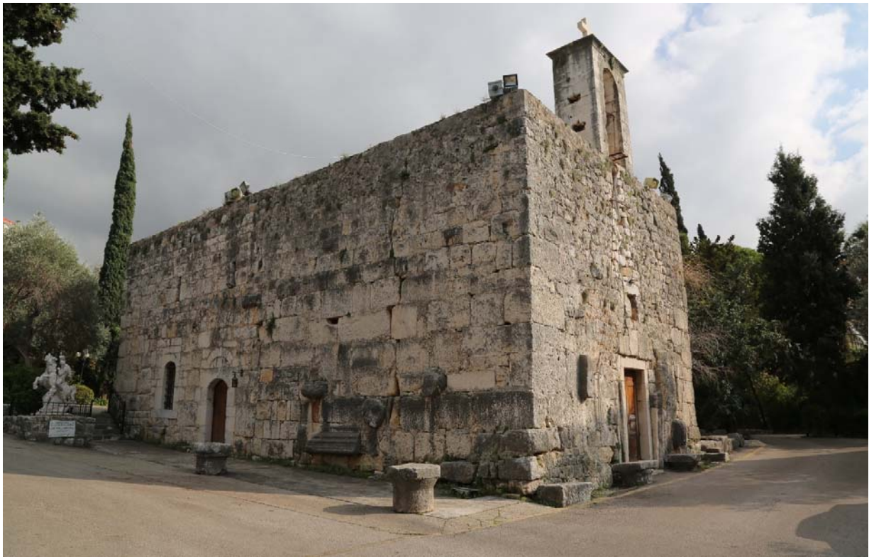
Figure 42: Saint Georges spolia church of Eddeh – Northern western corner
