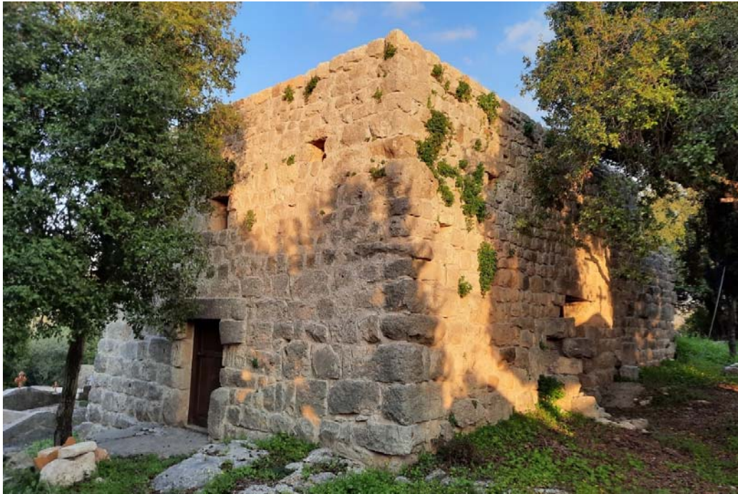
Figure 27: Saint Tekla spolia church of Chikhane - Southern western corner
