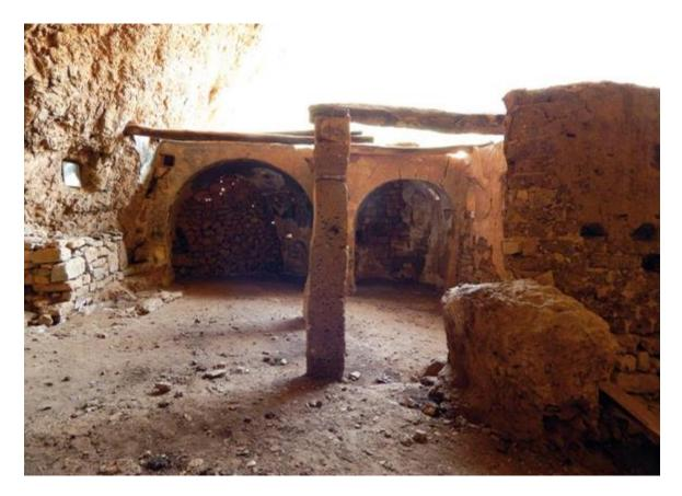
Fig. 111-Dayr al- Ṣalīb monastery, the two apses built with mode bricks.
