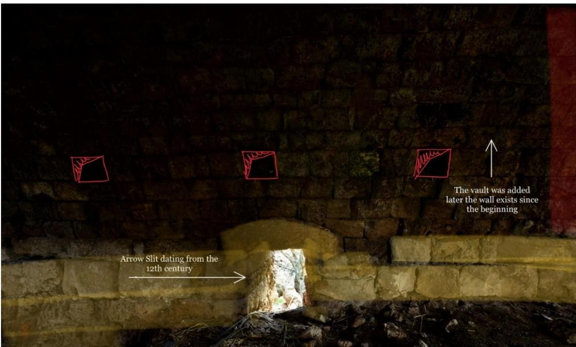
Fig. 21-Analytical view of the vault in the space 3.0.
