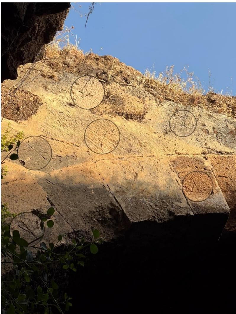
Fig. 62-Northern face of tower 4 showing Medieval assembly Marks.
