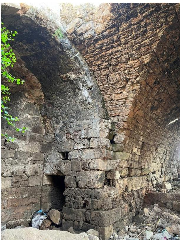
Fig. 23-Junction in between the tower 4.0 and the space 3.0 the vault was added later.
