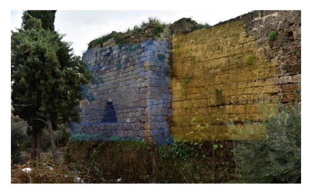
Fig. 45-Junction between wall 15 and the tower 16 on the eastern façade of the castle enceinte.
