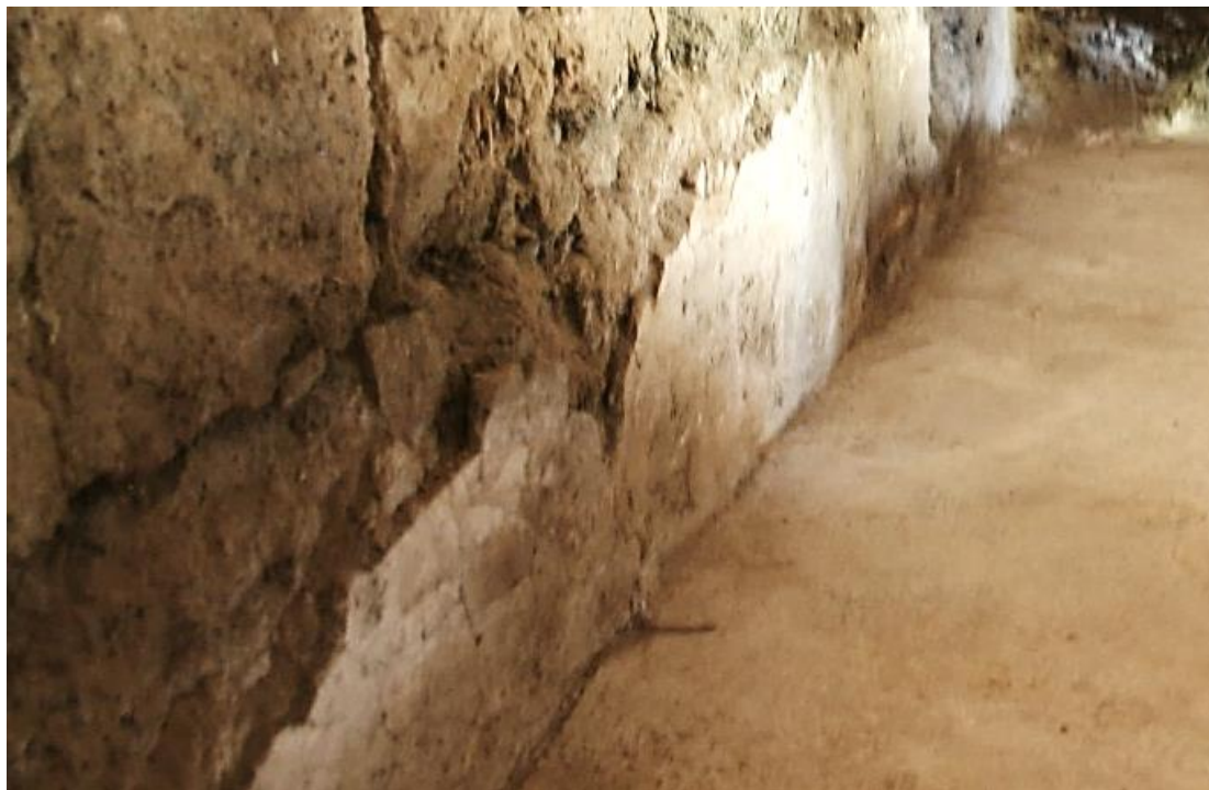
Fig 156. Remnants of layers of preparation of wall paintings, al-Ḥarfūsh, Philippopolis, Syria, (Photo: Osama Nofal, 2014).
