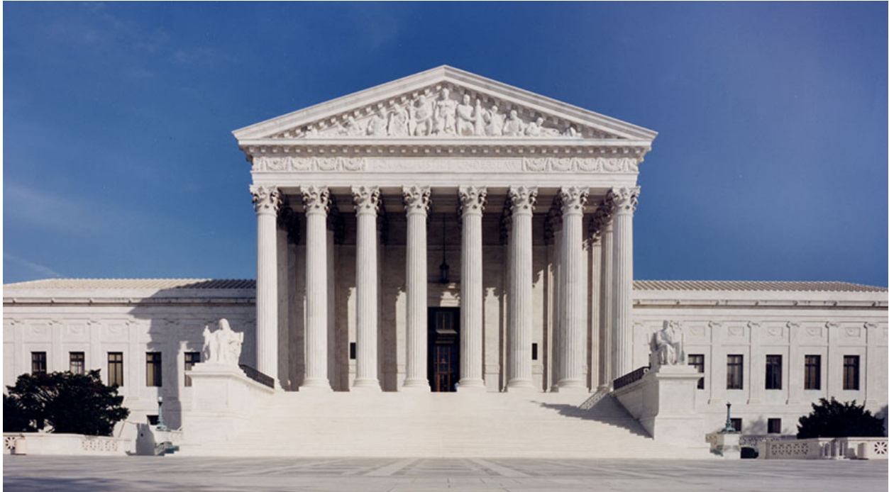
The building of the US Supreme Court in Washington DC 111
